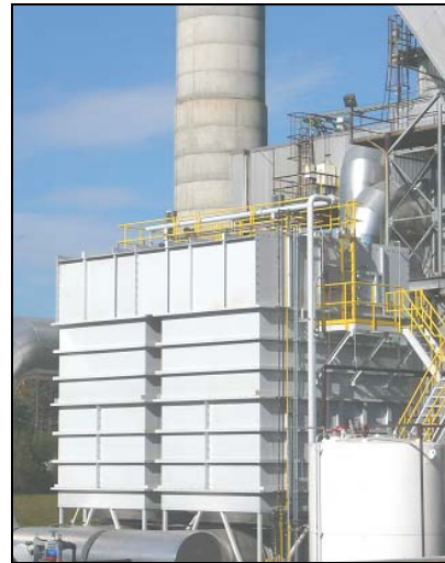
Figure 7: An installed two canister RSCR System on a 15 MW unit
